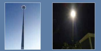
The Yard lights previously consisted of Metal Halide Lamps which consume about 1000W per lamp. With the direction of CMPort, HIPG Engineering Department decided to replace the old lamps with more energy efficient LED lamps which consume 420W of electricity while producing more light output whilst improving efficacy.
